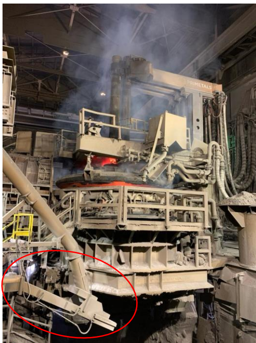
Alloy chute where operators add and push material into the ladle.
