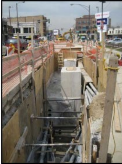
Figure 4 Vault Construction
