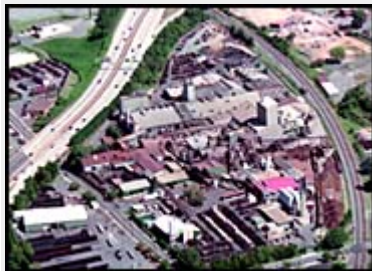
Cast Iron Foundry – Charlotte, NC
