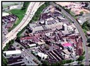
Cast Iron Foundry – Charlotte, NC
